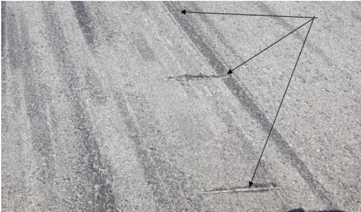
Figure 3: Slash marks caused by the propeller blades striking the runway surface
